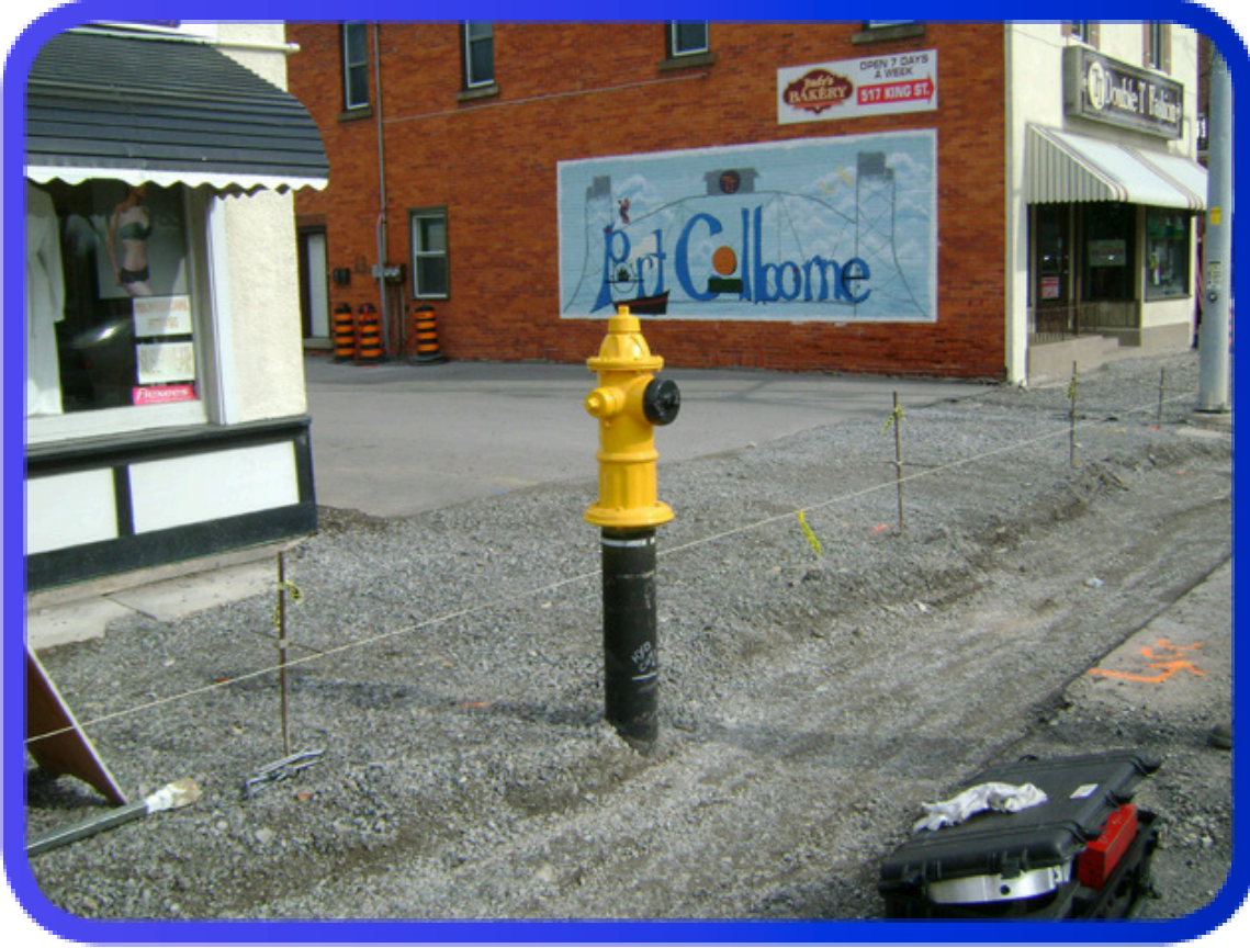
6' Hydrants installed on Main that varied from 2' to 3' below grade
