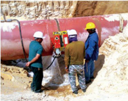
The Trav-L-Cutter can cut vertically, horizontally or anything in between
