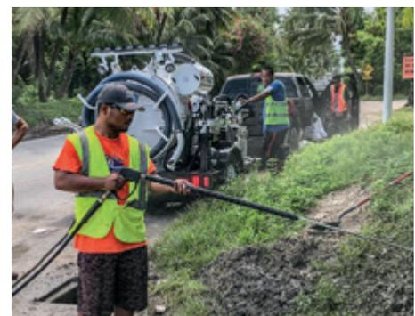
The included pressure washer system is ideal for cleaning valve boxes and covers
